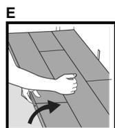
**E) Separate the whole row by carefully lifting-up and release the whole row.** Fold up the row and release the whole long side.
